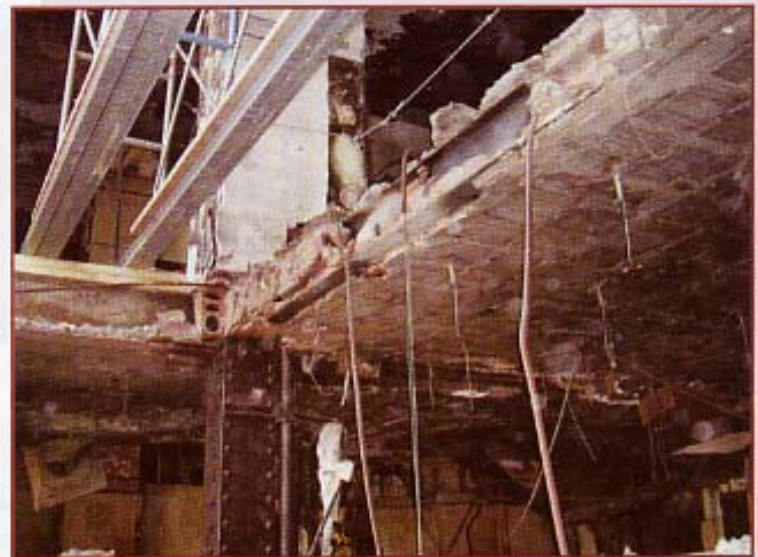
Figure 5. Flat arch tile floors in 90 West Street.
