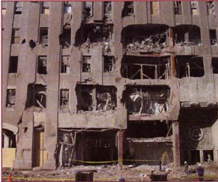
Figure 2. East elevation of 140 West Street.
