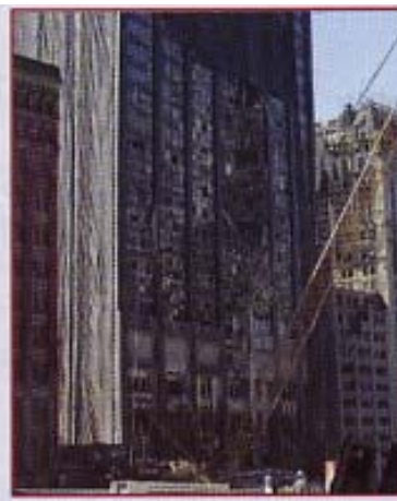
Figure 3. North elevation of 130 Liberty Street, Bankers Trust.
